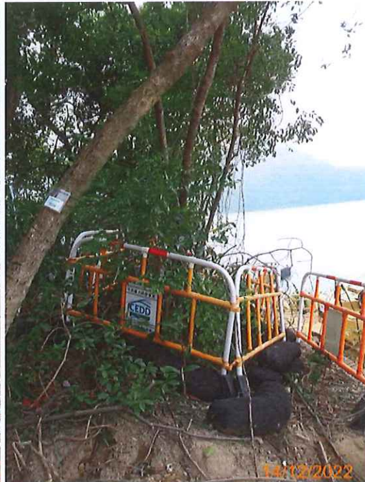
8: Protective fence sealed by sand bag
